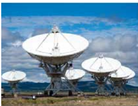
Figure 2.86 Energy reflects off of the parabolic reflector and is collected at the focal point. (credit: modification of CGP Grey, Wikimedia Commons)
